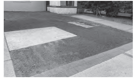
New soil is added to the landscape area and raked prior to planting.
